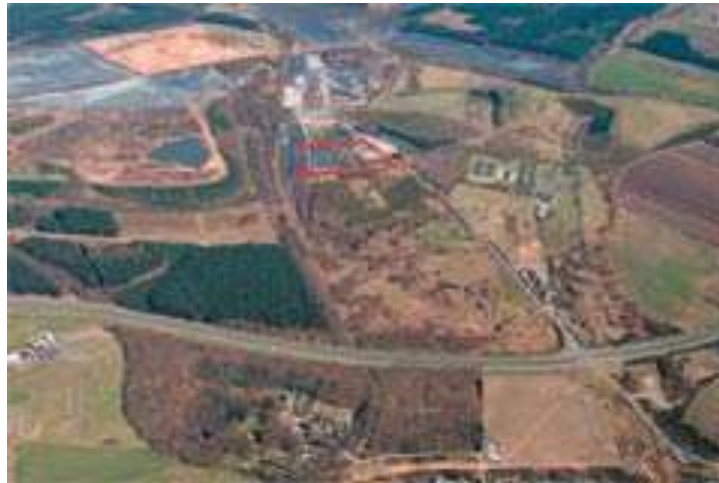
Figure 1.1e Aerial View of Proposed ERF Site
