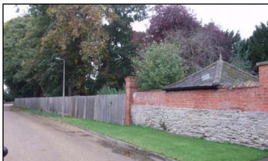
The lias boundary wall around the Old Hall in North Collingham gives way to a close boarded fence that could be improved
