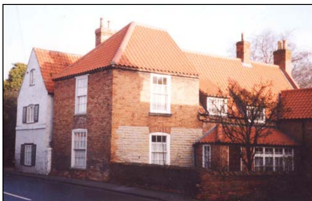
A part lias and part brick building, note the use of brick quoins and window headers
