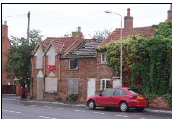
Row of vacant and dilapidated cottages on High Street
