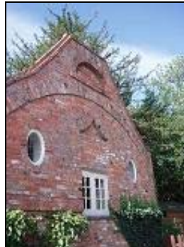
The Dairy on Gainsborough Road, associated with The Hall, is a simple vernacular building, but distinguished by interesting decorative detail on the gable end
