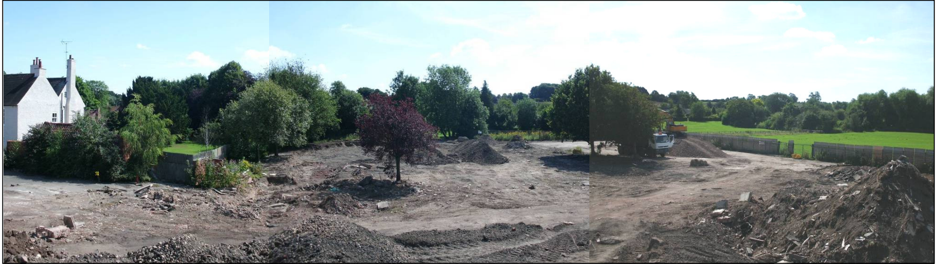
Plate 4: Composite panoramic view of the E side of the site, from a vantage point at the centre.
