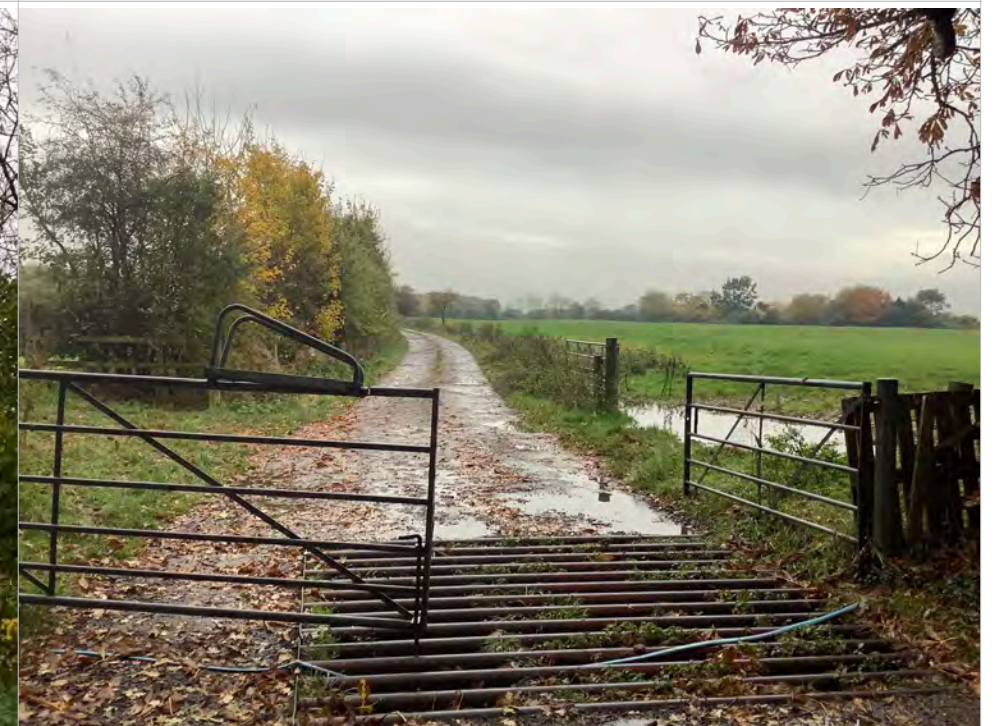
PHOTO 6: Existing access track to New Radley Farm in the northern section of the site. Note already compacted stone road surface.
