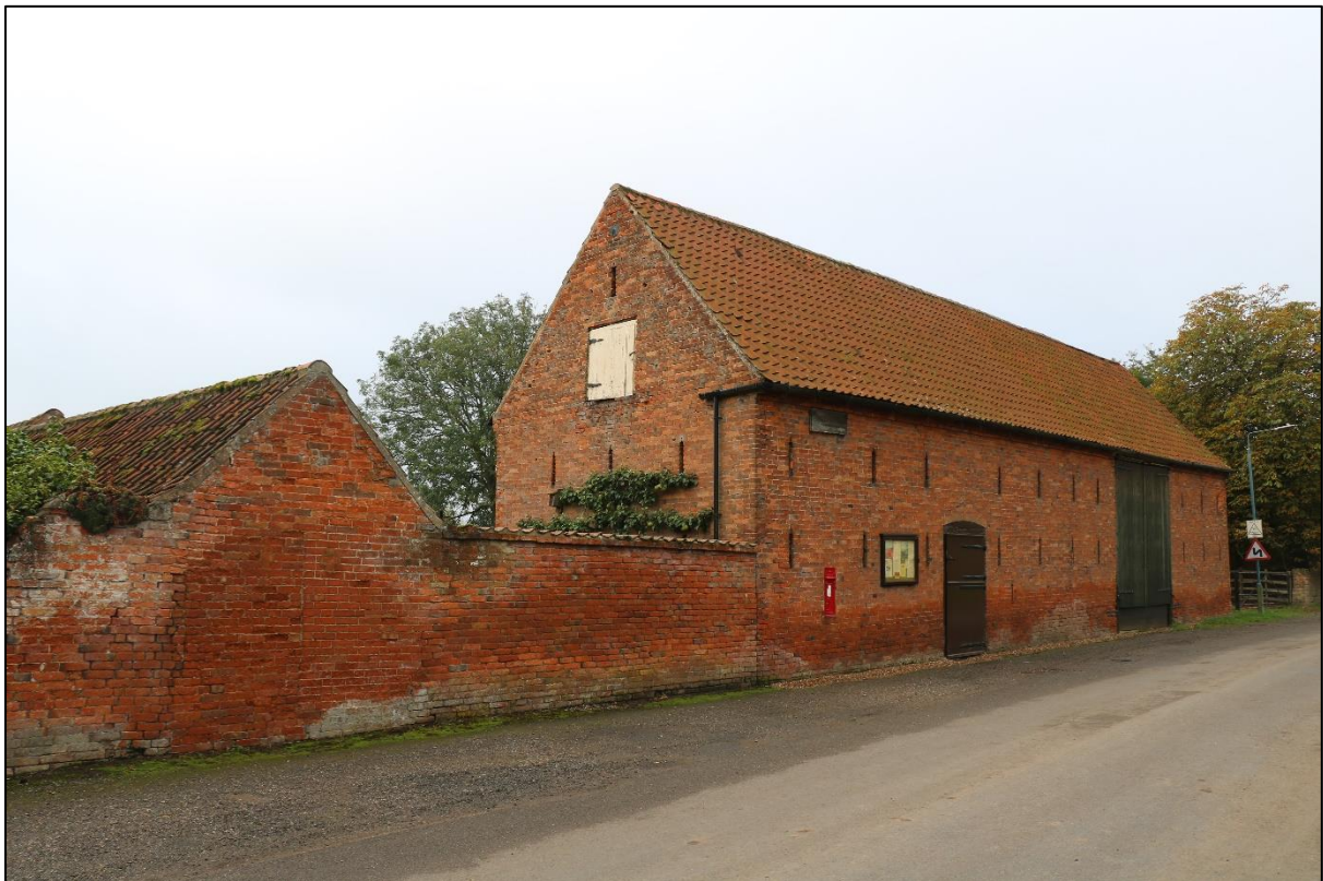
Figure 8 Barn at Halloughton Manor Farm viewed from the road side
