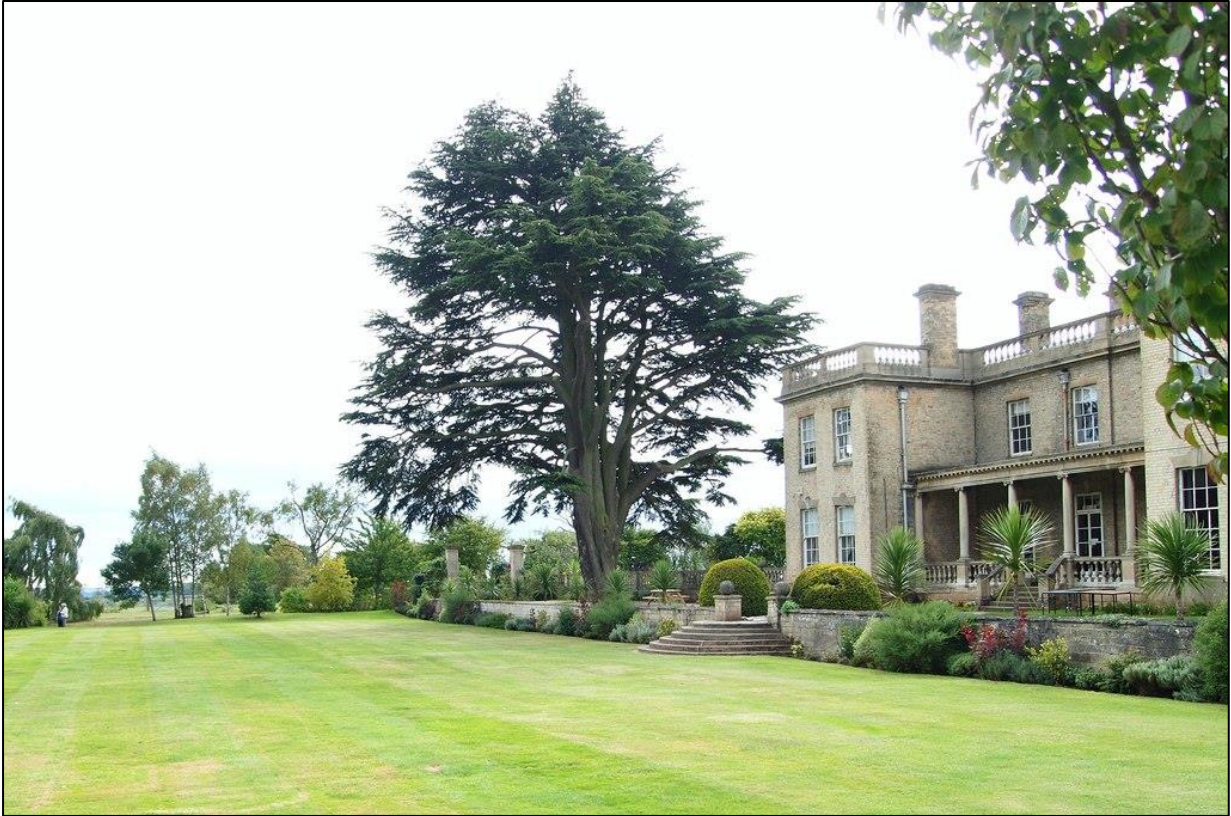
Figure 14: Brackenhurst Hall, east elevation PHOTO © DAVID HALLAM-JONES (CC-BY-SA/2.0)
