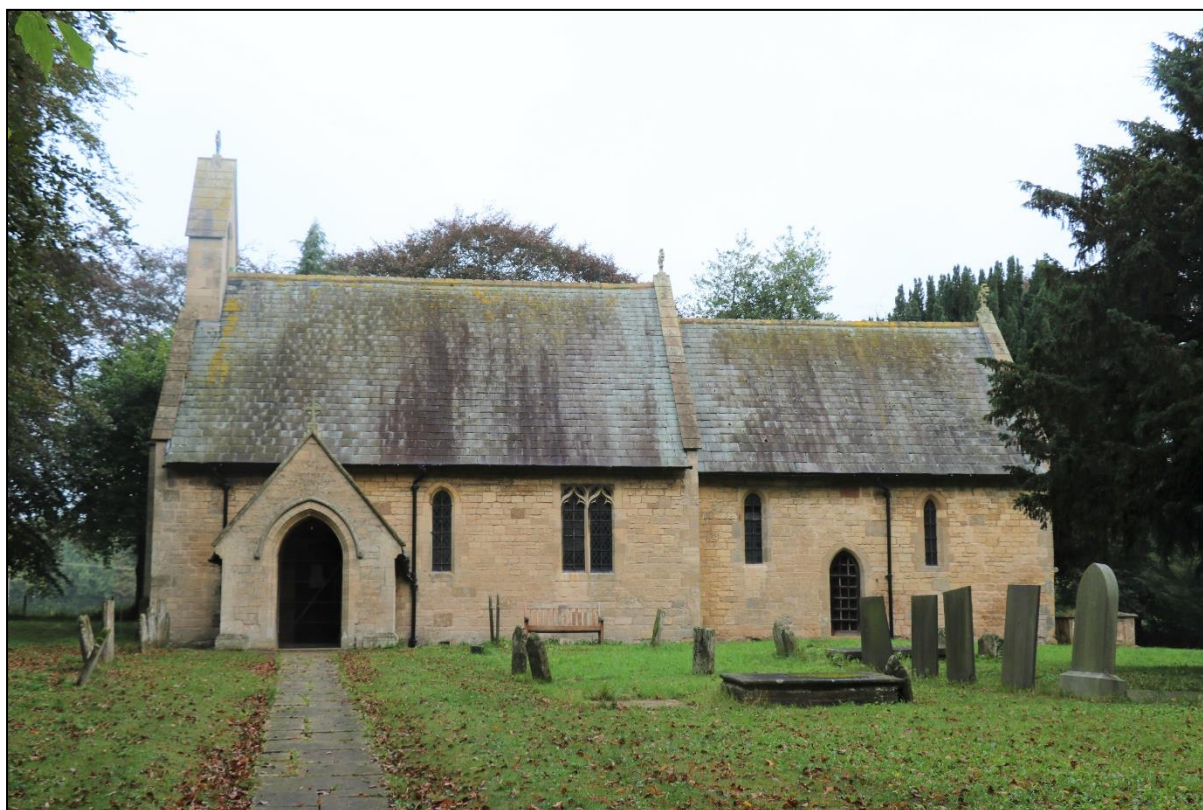
Figure 54: Church of St James viewed from the south
