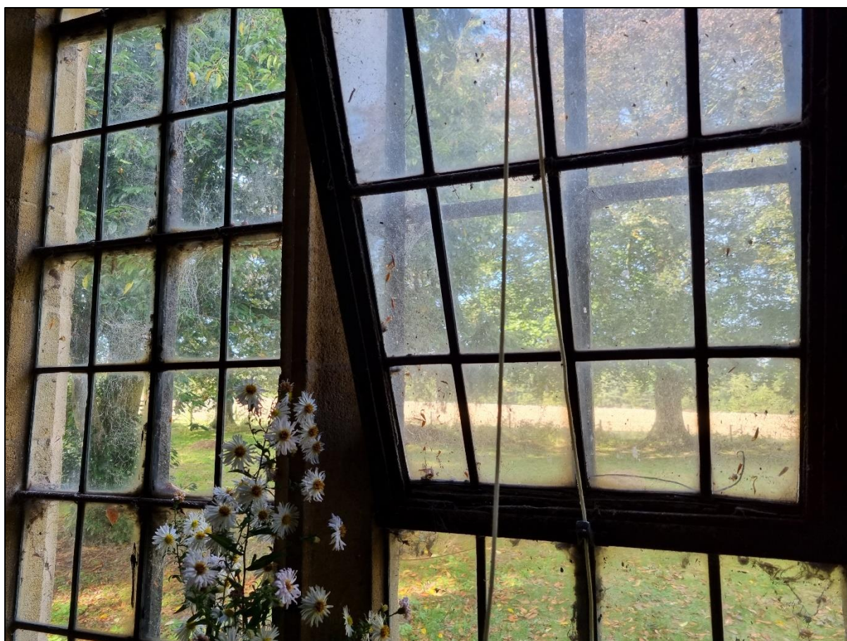
Figure 56: View north from within St James Church
