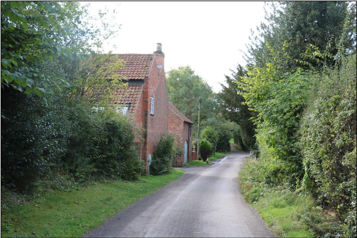
Figure 27: View along Bridle Farm Road within Halloughton Conservation Area
