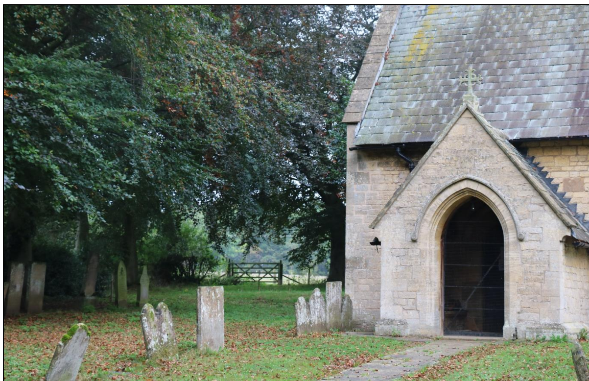
Figure 55:View north from within the southern part of the graveyard
