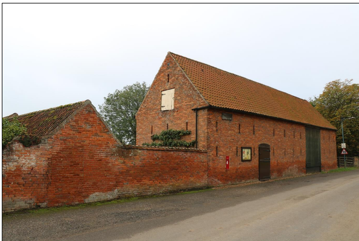
Figure 45 Barn at Halloughton Manor Farm viewed from the road side
