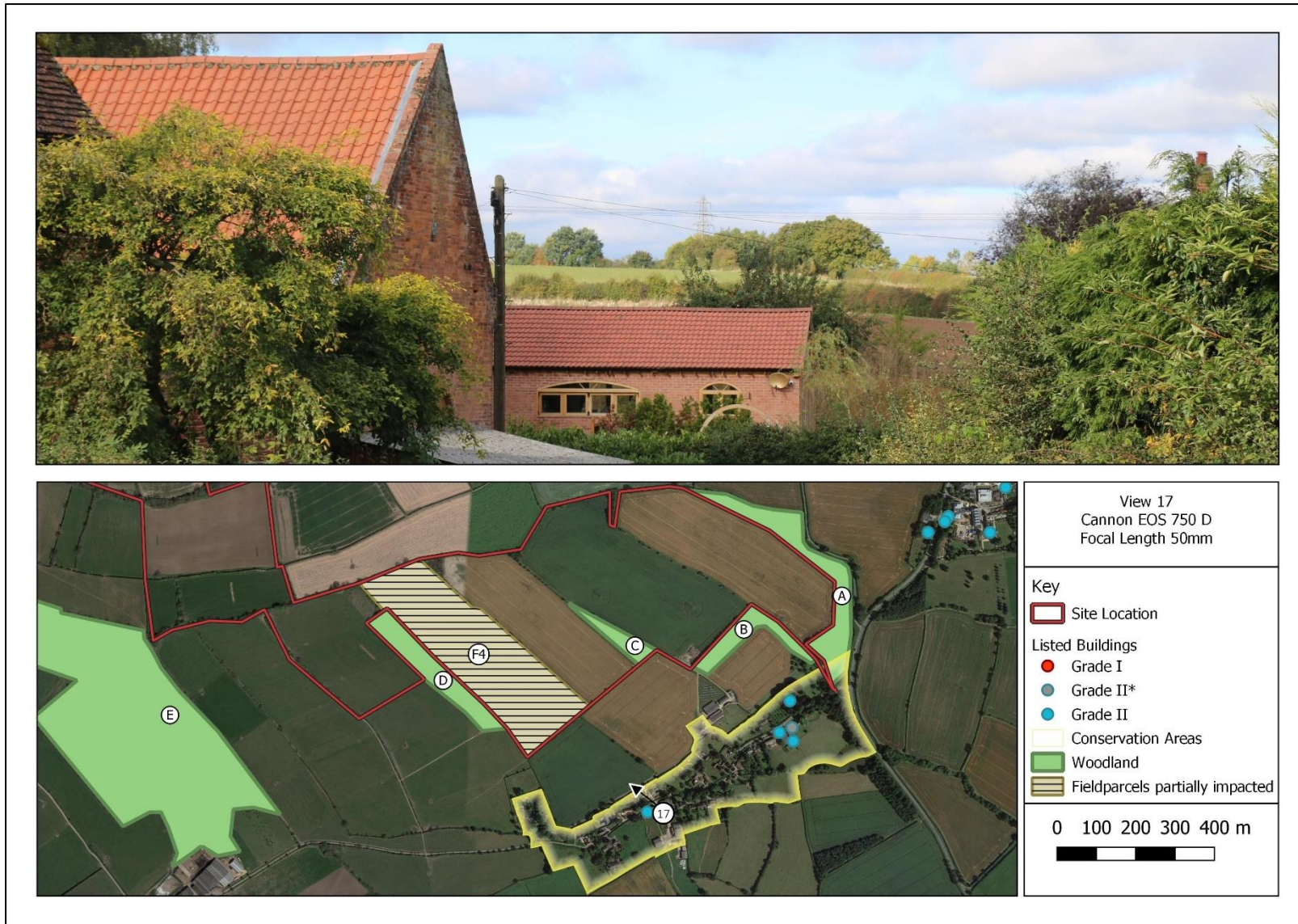
Figure 84: View 17 from within the Halloughton Conservation Area featuring the eastern gable-end of the Grade II listed Barn at Bridle Road Farm, featuring the Site behind
