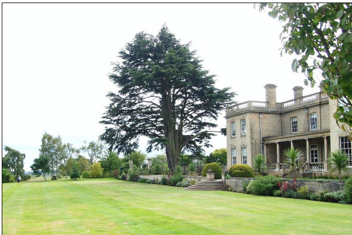
Figure 36: Brackenhurst Hall, east elevation PHOTO © DAVID HALLAM-JONES (CC-BY-SA/2.0)
