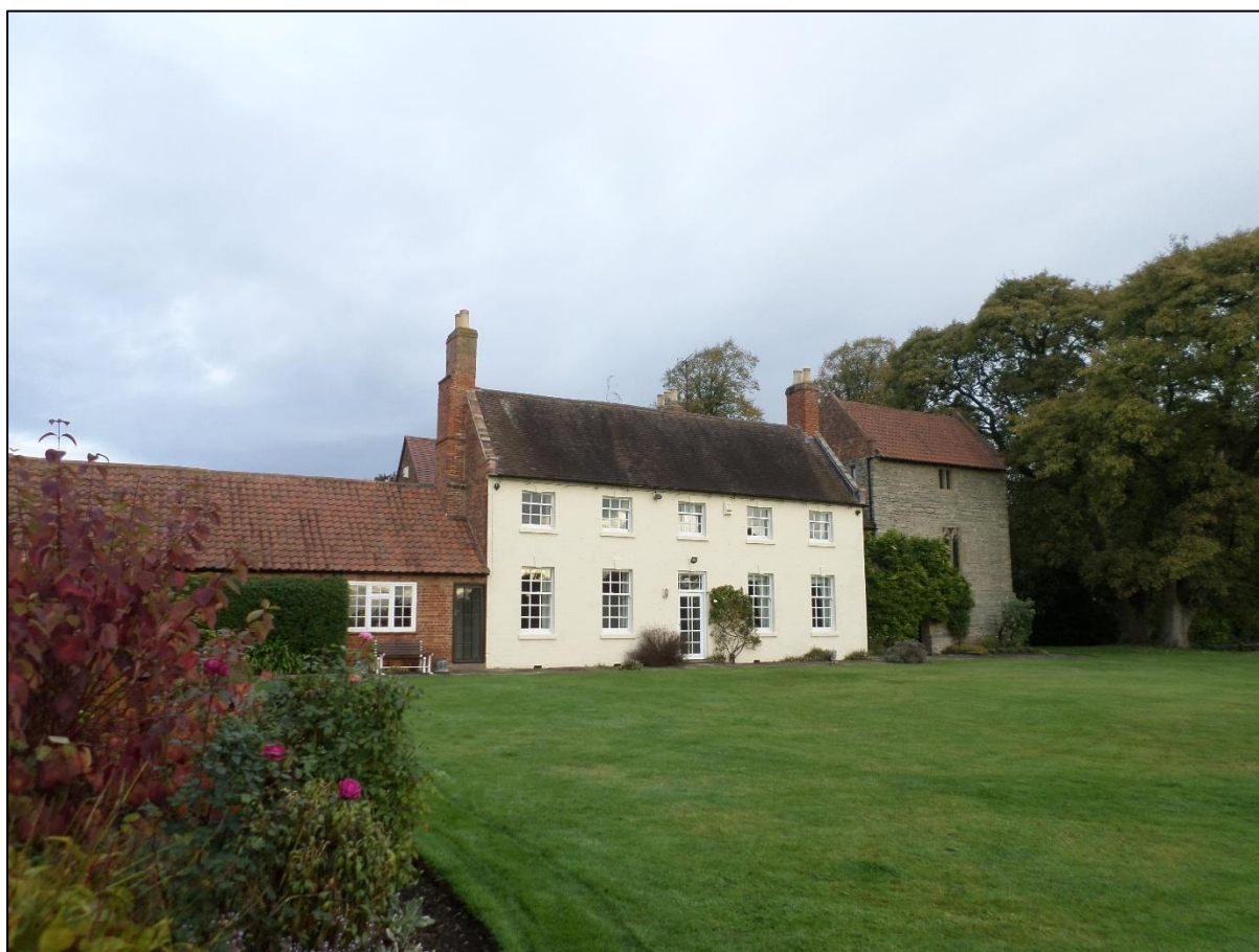
Figure 44 Rear elevation of manor
