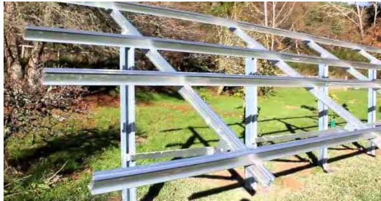
Figure 3.3: View of typical ground mounting system
