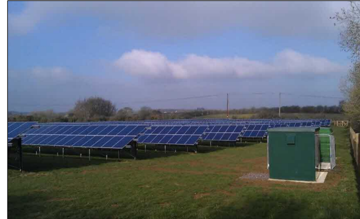
Figure 3.2: Ground mounted PV panels and transformer
