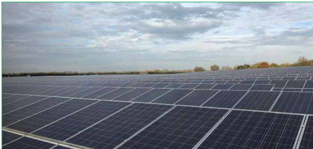
Figure 10 - Typical View of Arrays with Joints which Distribute Runoff
