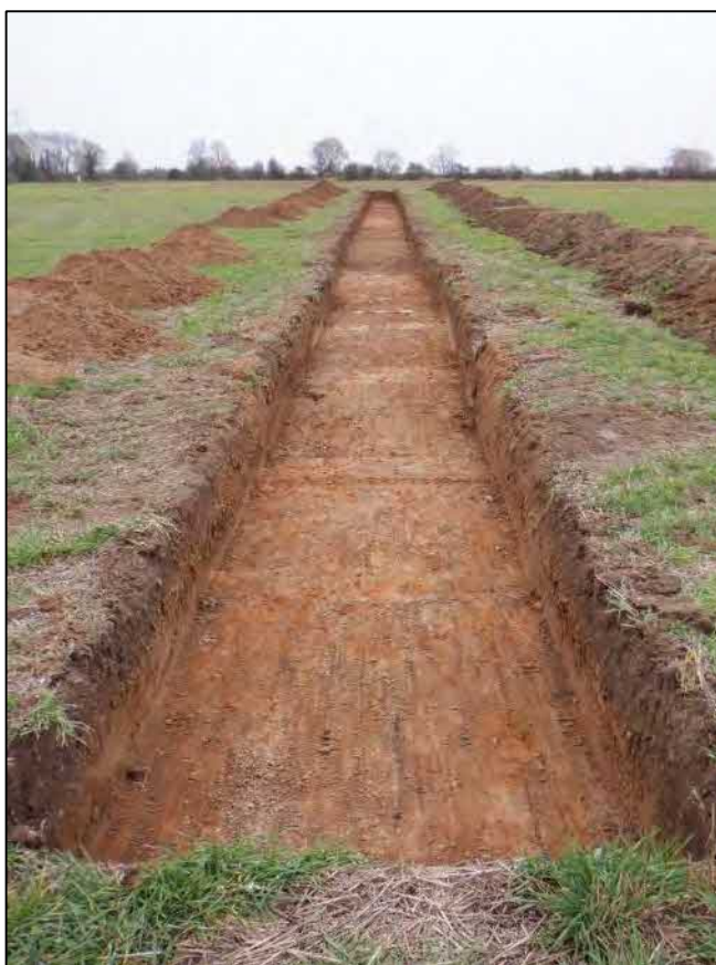
Plate 3: Trench 2, looking northeast
