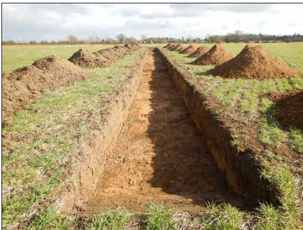
Plate 61: Trench 25, looking east.
