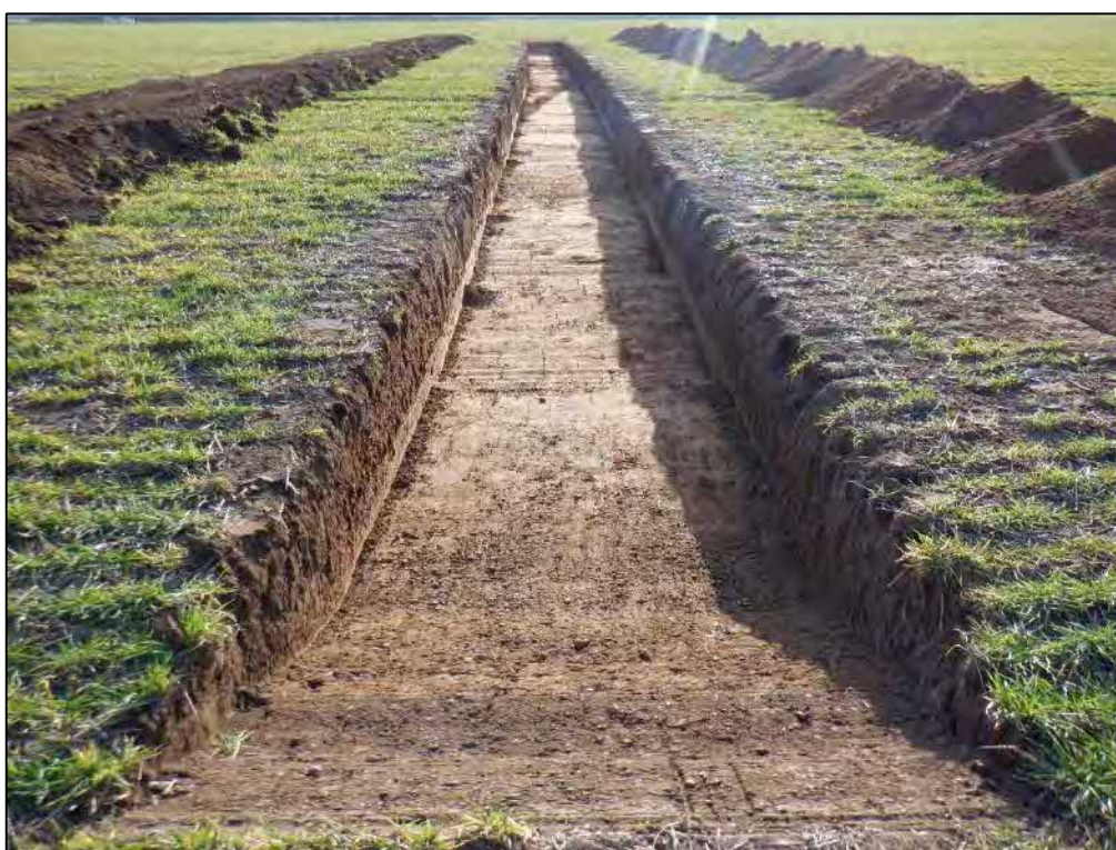
Plate 32: Trench 14, looking northeast
