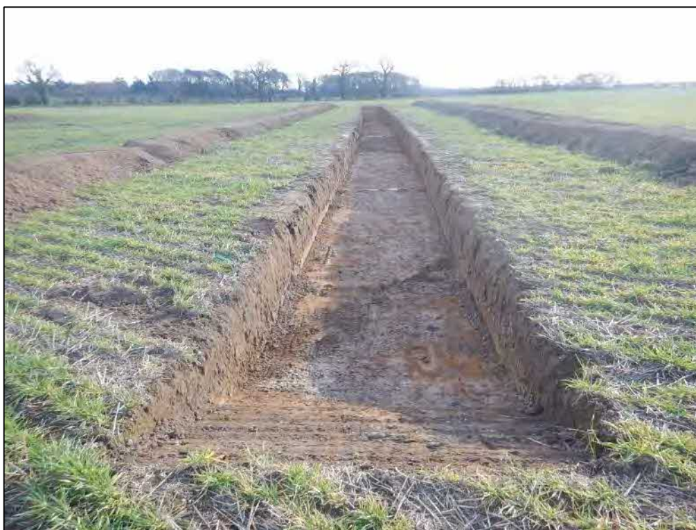
Plate 49: Trench 18 looking south.
