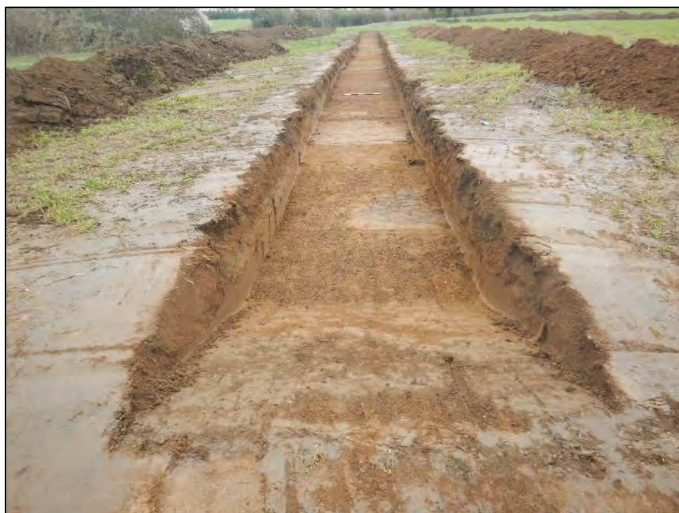
Plate 128: Trench 57, looking north east.
