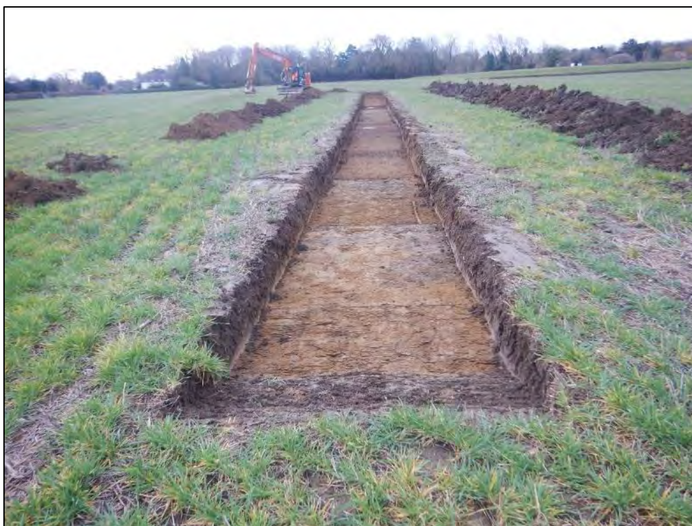
Plate 89: Trench 42, looking southeast
