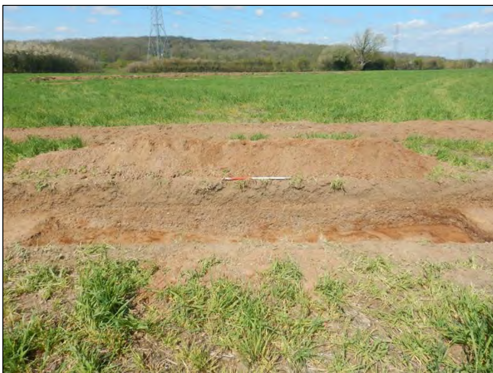
Plate 168: South facing of [73002]
