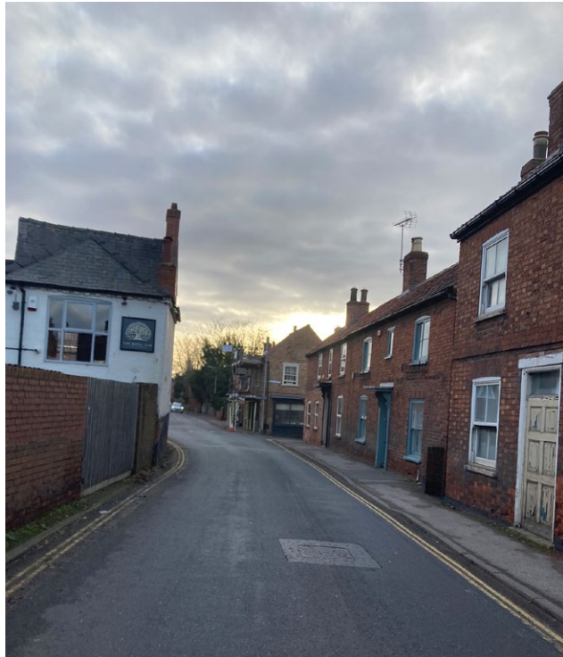
Figure 22: Footways in the historic core are often only on one side or are too narrow.
