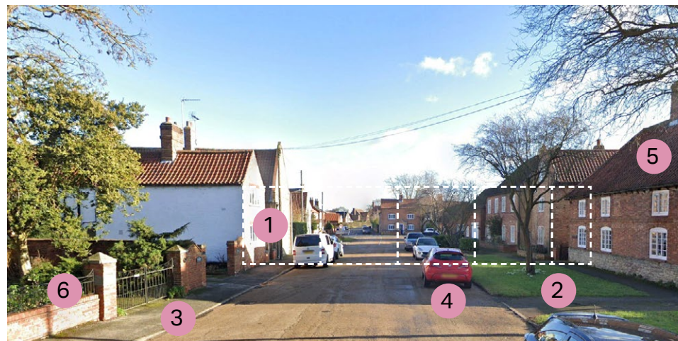
Figure 08: Looking east along Low Street.
