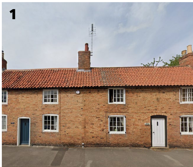
Red brick and pantile joined-cottages with no set-back
