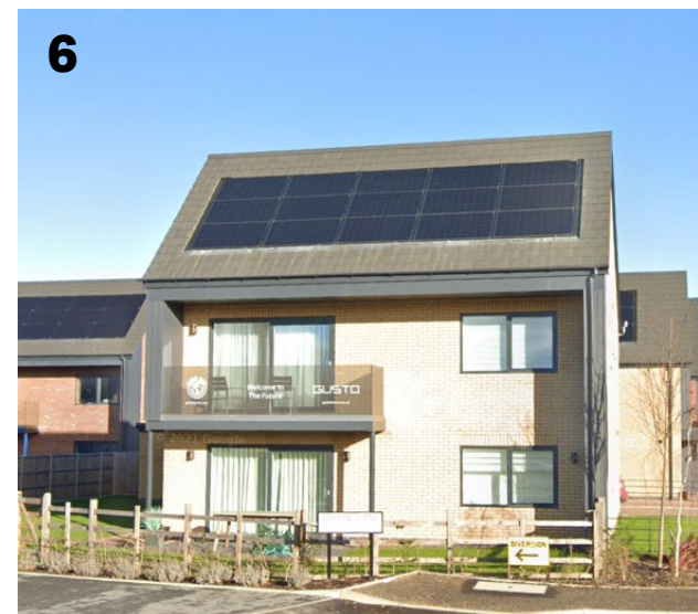
House in the most recent development of Collingham including solar panels
